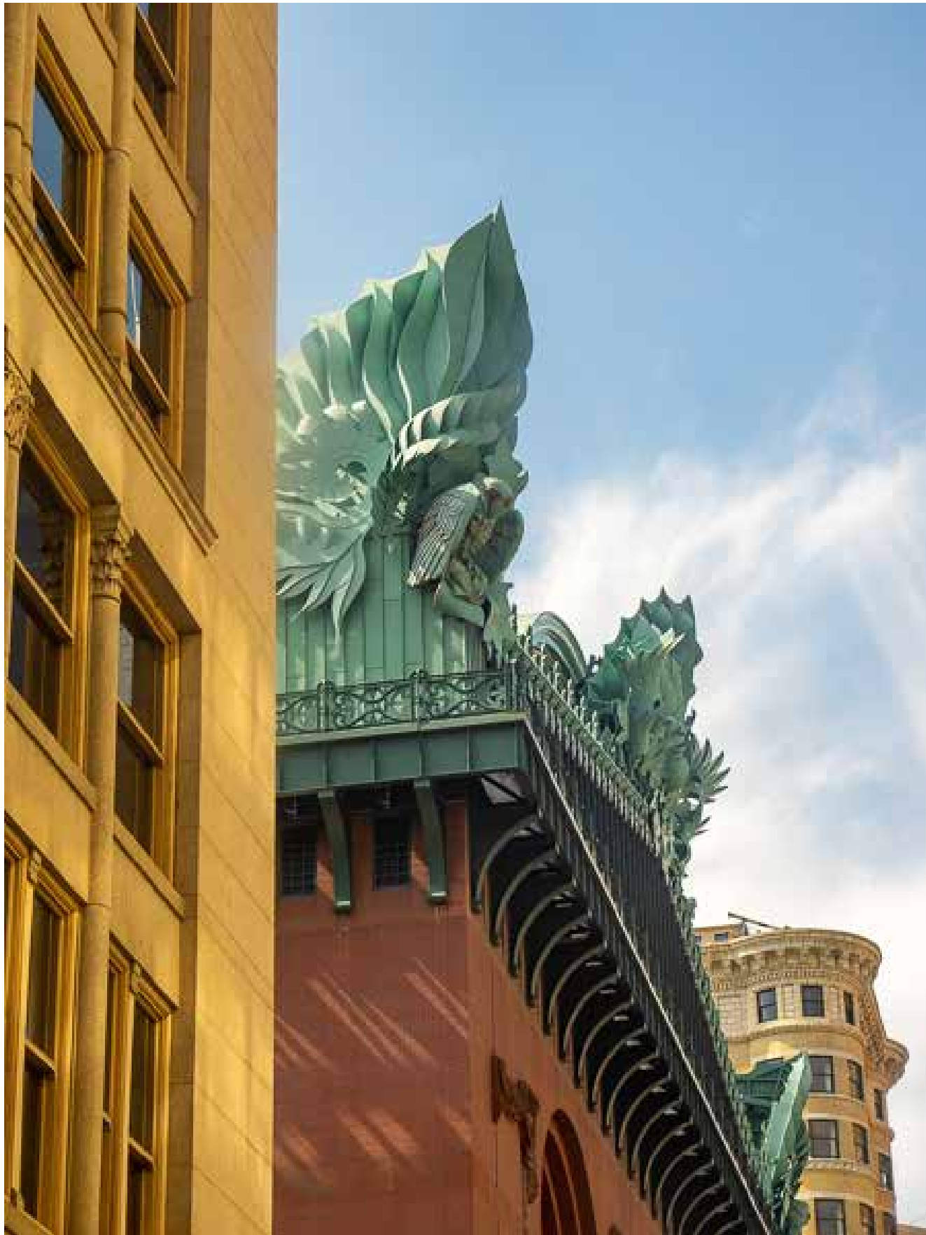
Gargoyles on top of the Harold Washington Library watch over the tracks.
