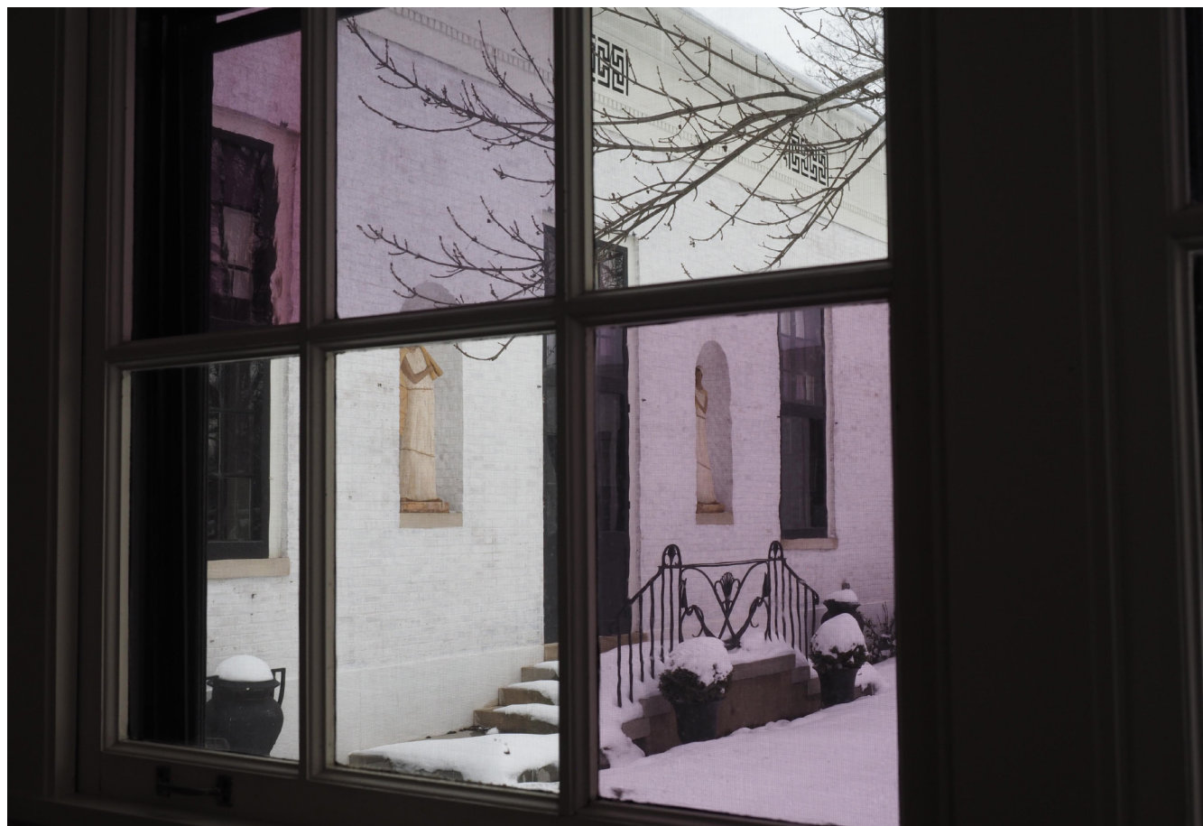
Amber glass, a unique detail of the original windows in the Clow house, lends a subtle filter to the light that streams into the home.
